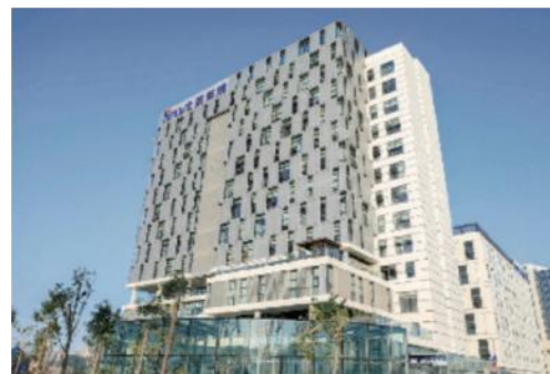
INVT Guangming Technology Building
