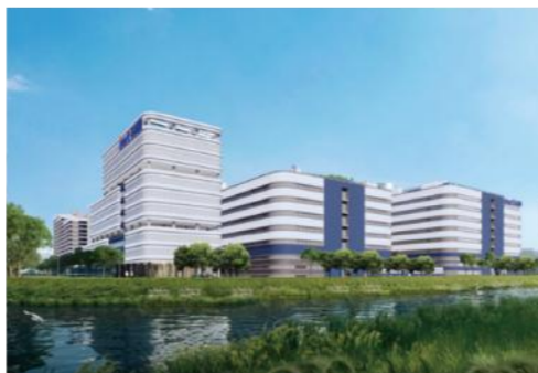
Zhongshan Industrial Park (Building)
